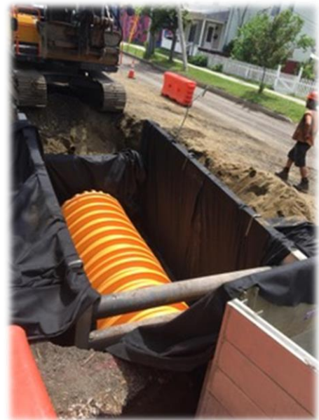
Figure 1. Park Street Infiltration Installation
